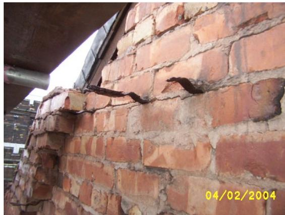
Corroded thick metal ties where outer leaf has been dismantled
